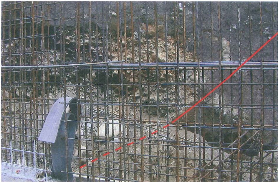
Figure 5. The gravel horizon thrust onto the sand and clay horizons, and the gravel bed dragged by the Chi-Chi earthquake rupture forming an anticline in the hanging wall.
