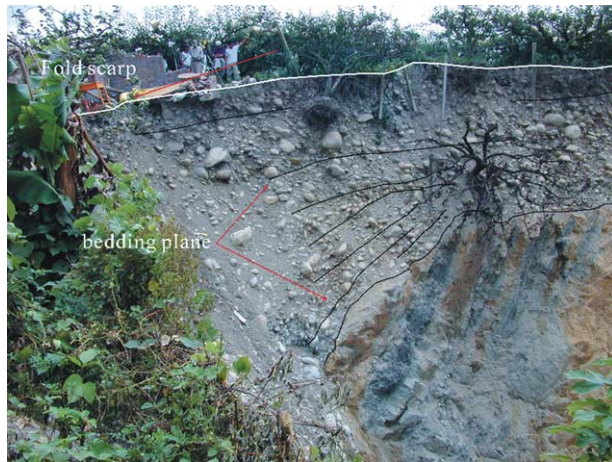
Fig. 7. Topographic expression of the pear field exhibited a folded scarp produced by the earthquake. Note that the gravel bed of terrace deposits on the fold scarp forms a wedge shape and the upper bed displays less inclination compared to the lower bed which dips 60^\circ . Obviously, the gravel bed has progressively tilted over time. This site is 50 m apart from Fig. 8.
